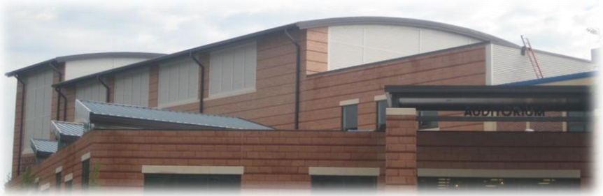
Figure 5: Barreled Auditorium Roof
