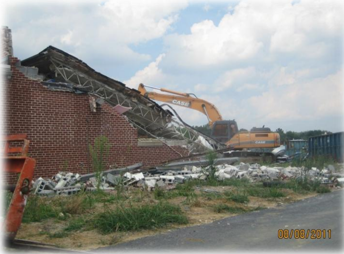
Figure 4: Demolition during Phase 4
